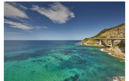
Sea Cliff Bridge, Clifton
